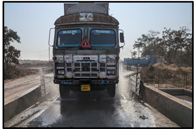
Wheel washing system at Jagannath OCP
