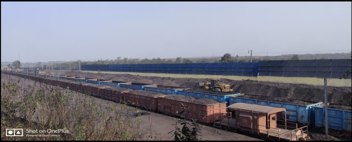
Wind barrier at siding no.2, Samleswari OCP
