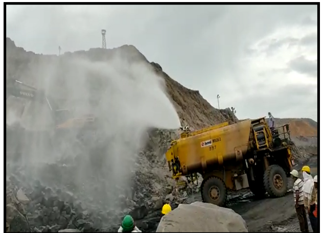
Robotic nozzle, retro fitted on 28KL mobile water taker Lingaraj OCP
