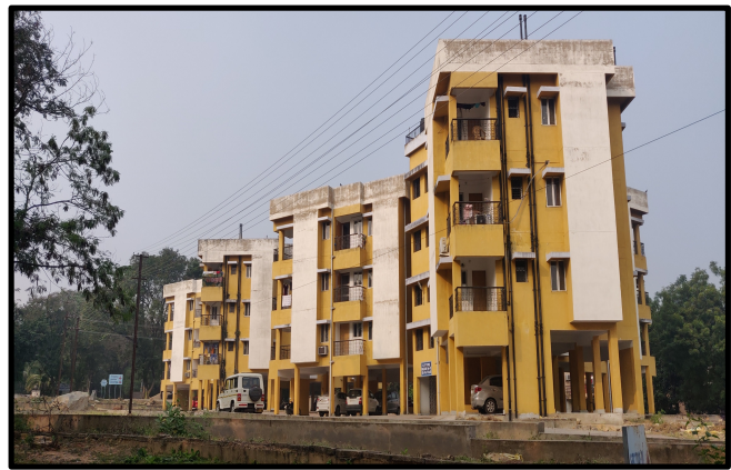
Employee quarters at MCL, Head Quarters
