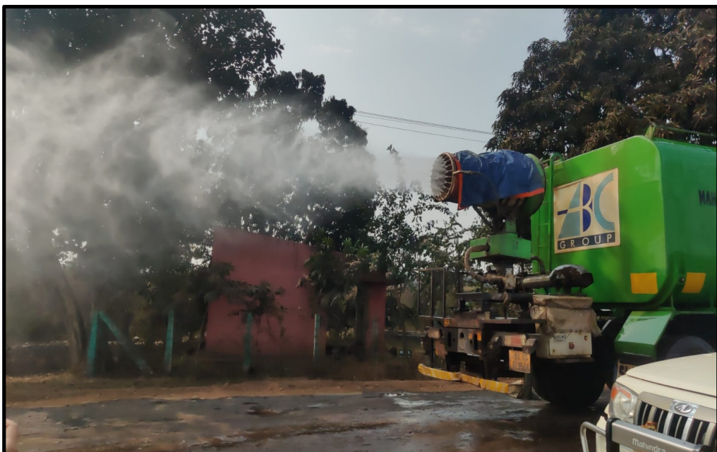
Truck mounted Fog cannons (40m throw) at Kaniha OCP
