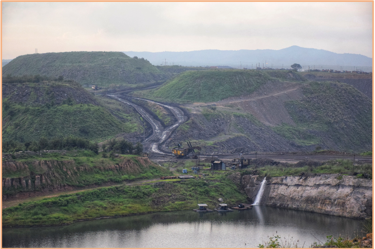
Mine sump of Ananta OCP
